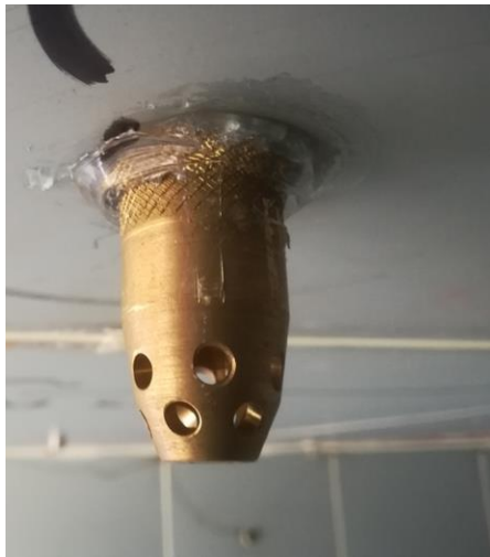
Nitrogen spray nozzle and nitrogen supply arrangement
